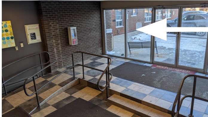
▲ View of existing front entrance to be reconfigured
